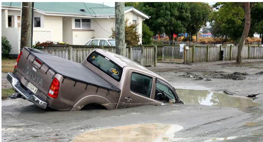
Gambar 1. Fenomena likuifaksi akibat gempa Christchurch, 2011 (Tonkin and Taylor, 2013)
